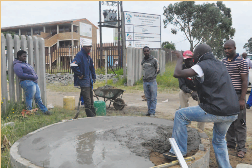
Intervention: Construction of a base for a Jojo tank in Ward 5, in Wesselton is underway to roll out jojo tanks in areas hit hard by water shortages.
