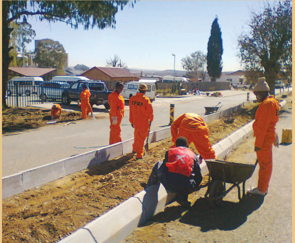
ROAD WORKS: Paving of the road island at Pertunia street became part of the road construction in Balfour.
